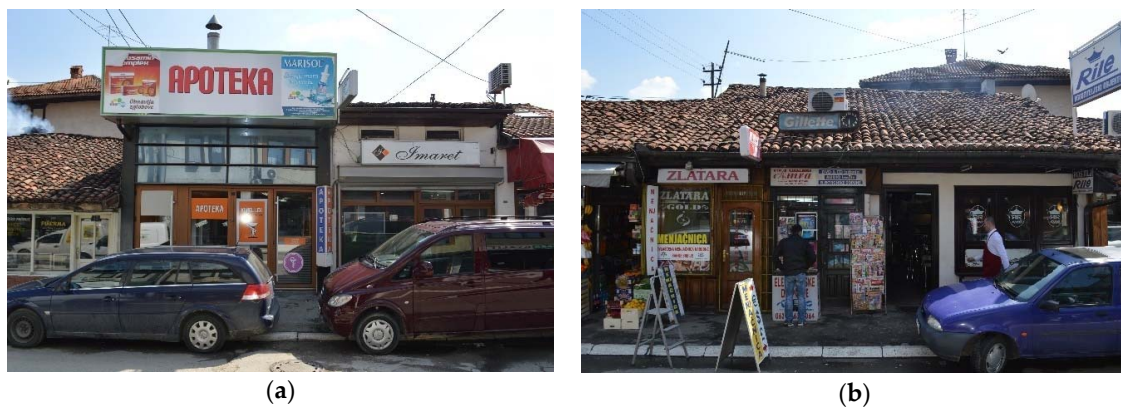
Figure 5. (a) Placing billboards in the historic center without any order; (b) new shop windows in a different color and material that are not suitable to the character of the historic center.
